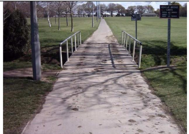
**Figure 19: Bridge with minimal rails and no approach barriers**
