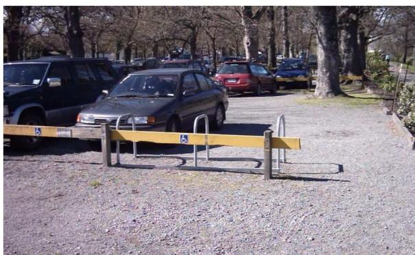
**Figure 29: Wrongly installed bike stand**
